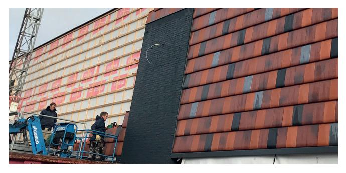
As well as creating outstanding roofscapes, Crest Nelskamp roofing tiles can also be used for facades/ walling or as often known as 'vertical cladding'. For technical clarification, BS 5534: the British Standard Code of practice for pitched roofs and vertical cladding, defines a wall as any surface at a pitch of 75 degrees or greater from the horizontal.
