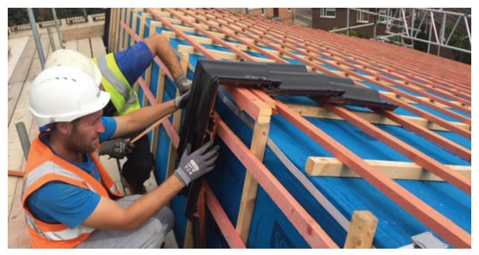
The Vertical Cladding/Mansard must be counter-battened, using graded tiling and counter battens in accordance with BS 5534.
